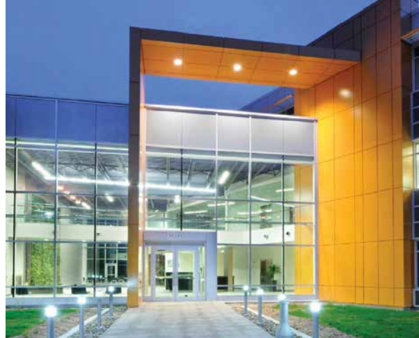
Provide good lighting at building entrances and along pathways.
