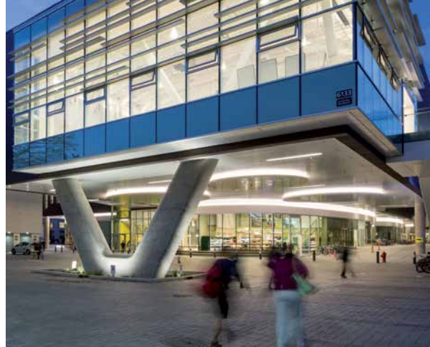
Emphasize building entrances and gateway moments with special features, clear views and ample lighting.
